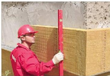
Rigid mineral wool can be an excellent substitute for polystyrene, owing to its moisture repellency and insect resistance. Photo: Rock-wool International A/S
