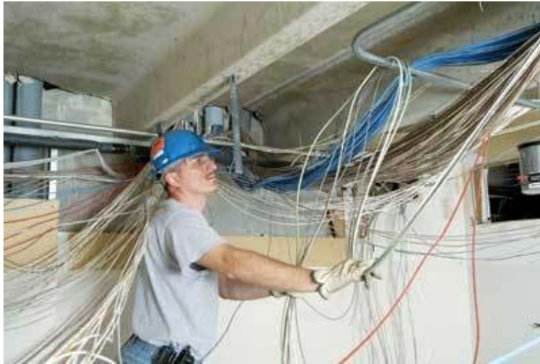
Removing abandoned wire and cable
