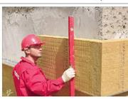
Rigid mineral wool can be an excellent substitute for polystyrene, owing to its moisture repellency and insect resistance. Photo: bodwool International A/S
