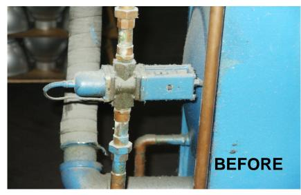
Solenoid Actuated ValvesEliminated "Flow Through "
