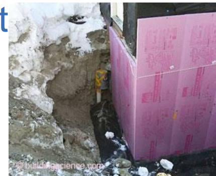
Building Science Corp.
