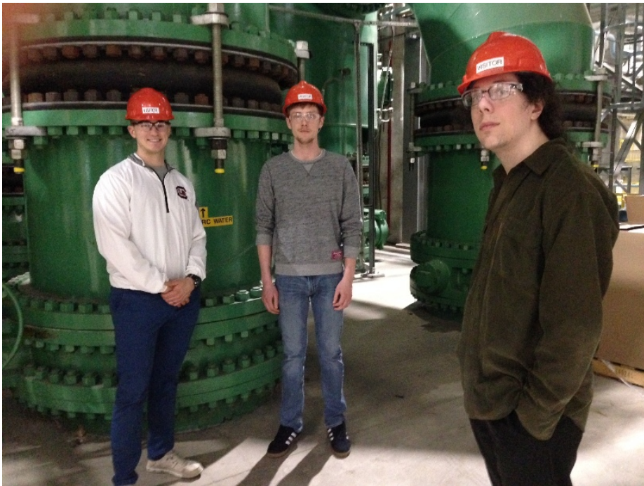
Forrest on left; these are the two water intakes at Calpine
