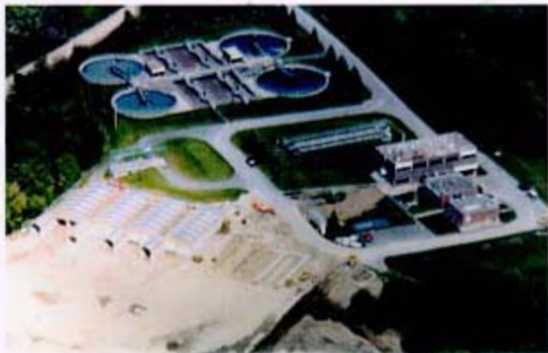
Hoosac Water Quality District Treatment Plant
